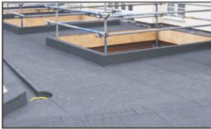
BITUMENOUS FELT LAYING
